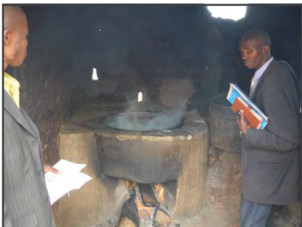
REF school director Henry Twinemasiko inspects the smoky kitchen's inefficient cookstoves. These have now been retrofitted to use fuel briquettes.
