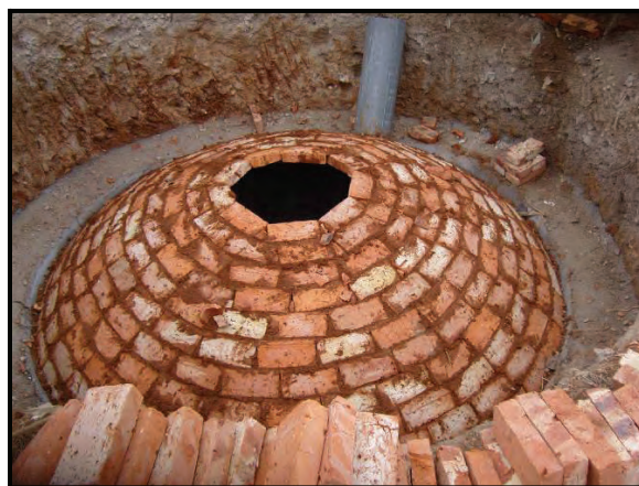
A biogas tank under construction
