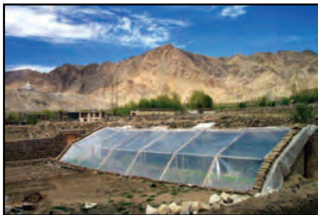
Passive Solar Housing, India
