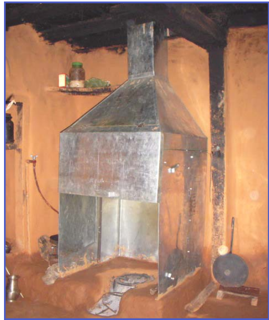
Intervention (smoke hood and stove improvement) in a household in Dhading District, Nepal
