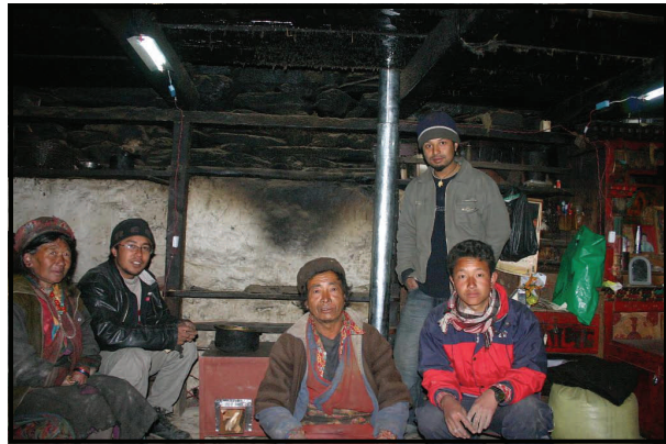
CSU stove installation in Nepal; January 2007
