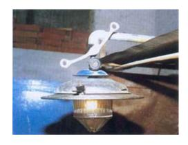
Biogas used for lighting Source: BSP/Nepal
